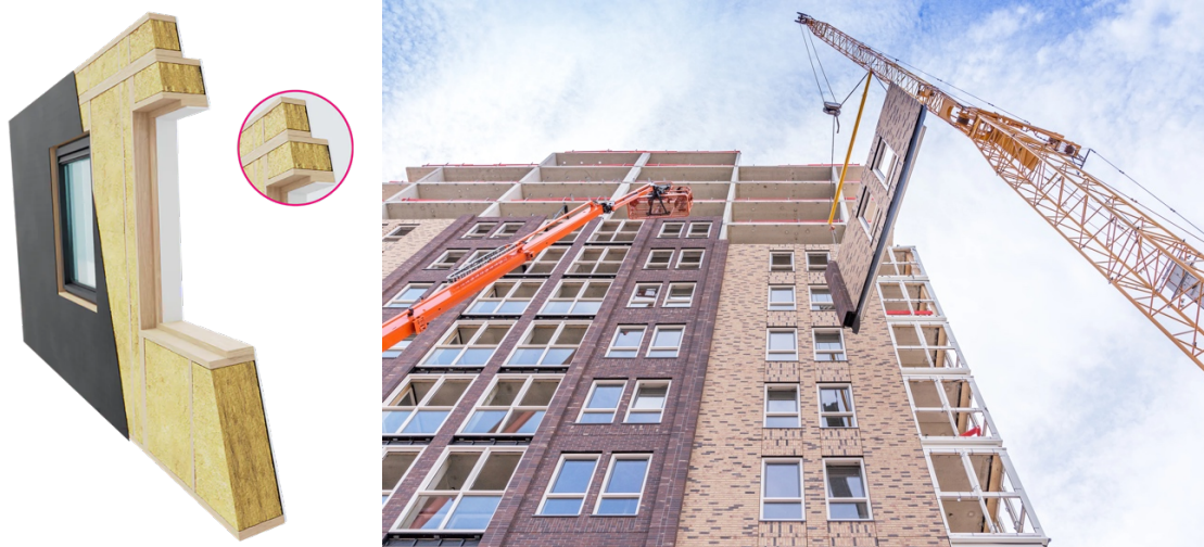
Figure 1. A typical prefabricated timber façade element section (left) and a real application (right, credentials: WEBO)
