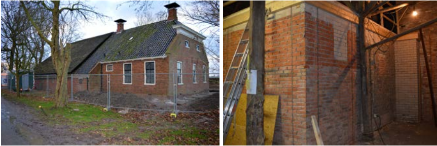
Figure 7.8: FDM CFRP strip retrofit. Westeremden, Groningen.
