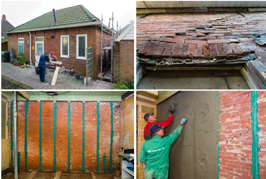
Figure 7.5: First commercial project using FDM CFRP strip and one-sided FRCM overlay hybrid retrofit. Usquert, Groningen.
