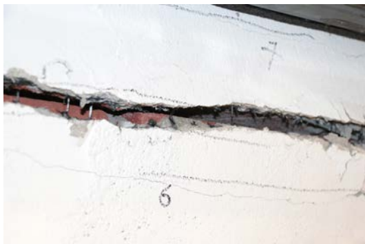
Figure 5.14: Close-up of the CFRP mesh rupture failure of FRCM-3 .
