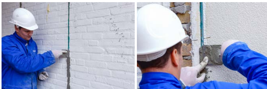
Figure 7.3: Closing the groove with the polymer modified mortar.
