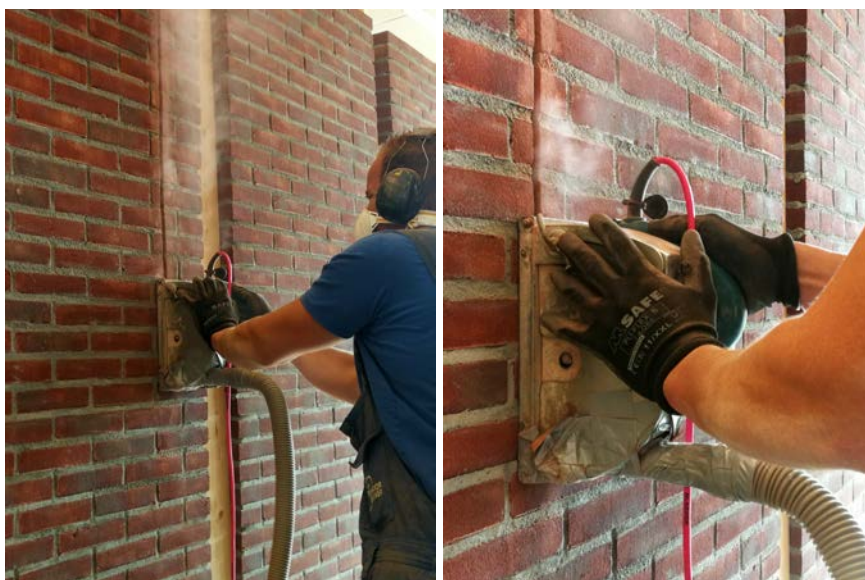
Figure 7.1: Deep groove cutting.
