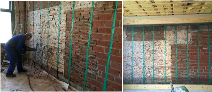
Figure 7.9: FDM CFRP strip and one-sided FRCM overlay hybrid retrofit (latter not shown). Appingedam, Groningen.
