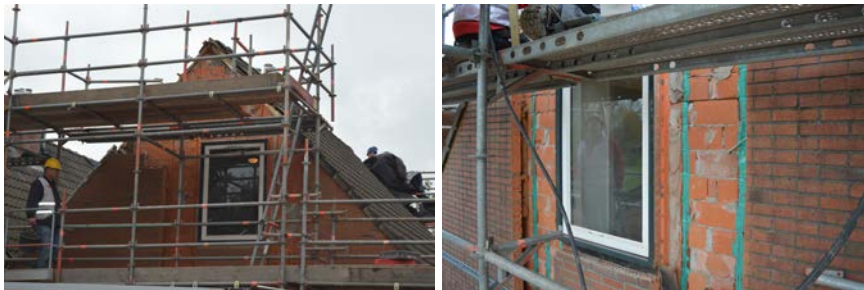
Figure 7.6: FDM CFRP strip retrofit on the inner leaf of the cavity wall, from the outside after controlled removal of the outer leaf. Zijldijk, Groningen.
