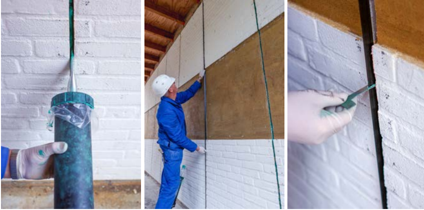
Figure 7.2: FDM CFRP strip installation.
