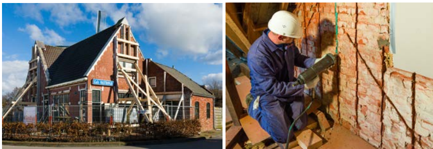
Figure 7.7: FDM CFRP strip retrofit on the top facade. Zeerijp, Groningen.
