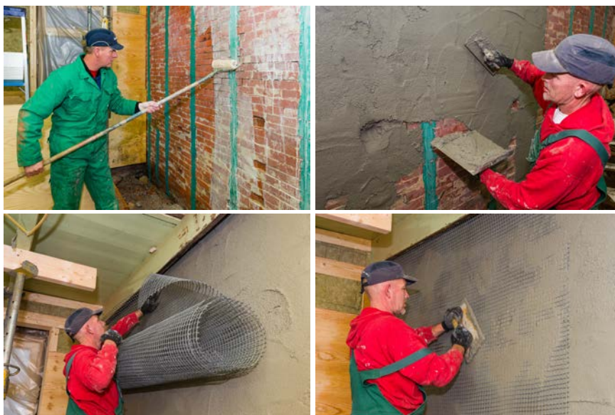
Figure 7.4: Single-sided FRCM overlay installation.
